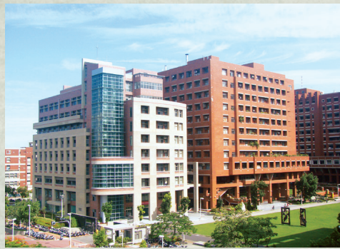
Department of Electrical Engineering
